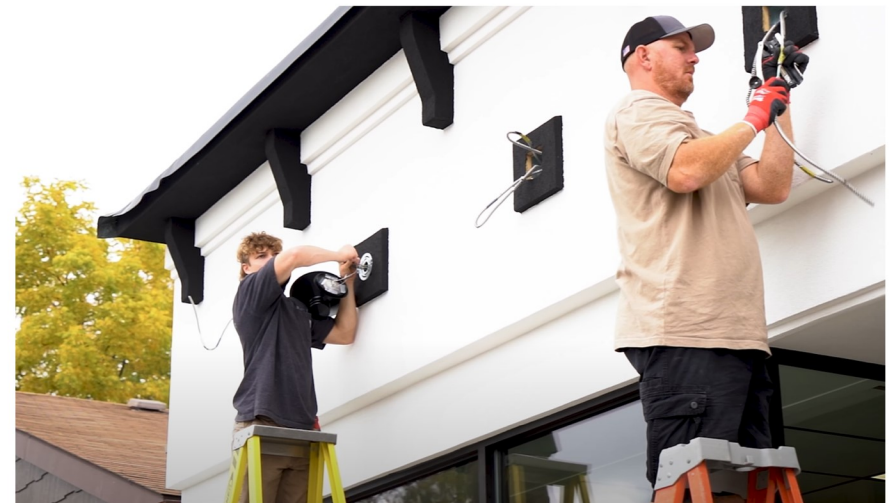
Top: Preliminary design rendering for 126 North Howard Street, as part of the DTR CDBG Application Bottom: Lighting being installed at 216 West Salem Avenue (Bob's Custom Trophies), as part of a grant awarded to renovate the existing storefront
